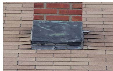
Failed Flashing
