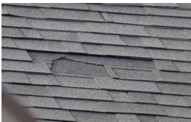
Missing Shingles
